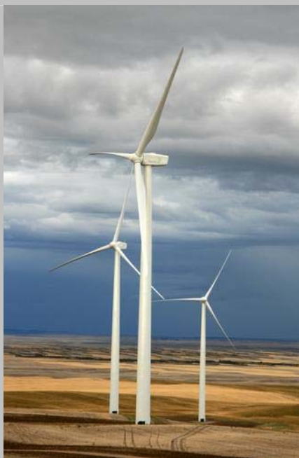
Wind turbines in Montana. Photo: Obel Kraus/NREL
